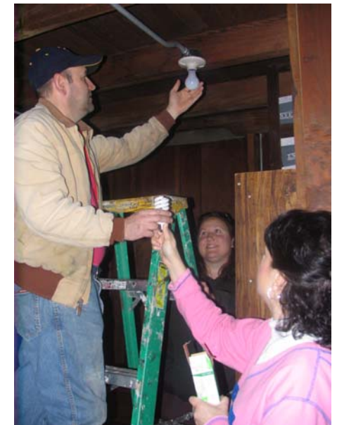
PMSS staff replace incandescent light bulbs with energy-saving CFL bulbs. Pictured left-to-right: James Smith, Cassie Robinson, and Faye Turner.
