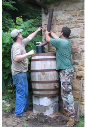
Randal Phleger and Eric Elrod install a rain barrel
