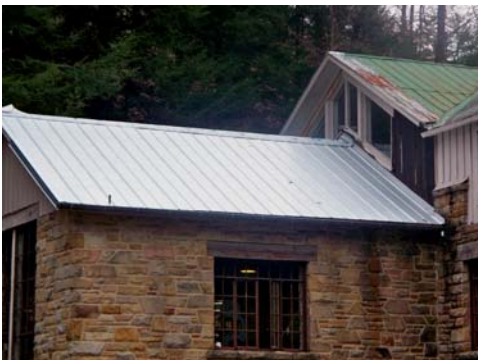
The west roof section on Draper Building is nearly completed.
