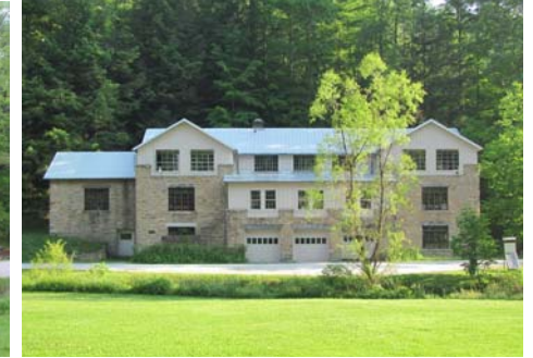
Draper Building – new roof
