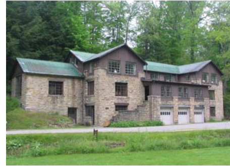
Draper Building – old roof
